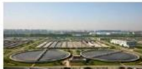
Sewage Treatment Plant
