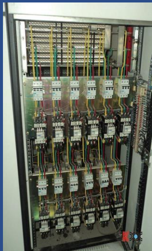
Contactor switching capacitor FC
